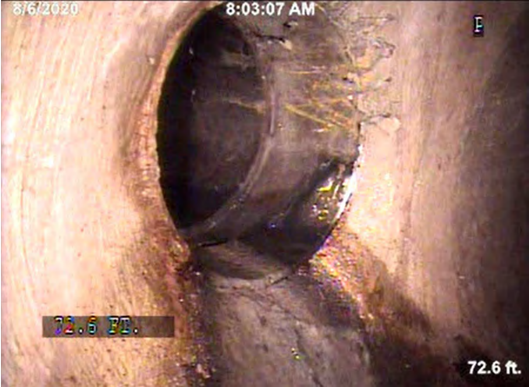
Figure 3B. Close up of illicit connection – note gray staining at the outlet
