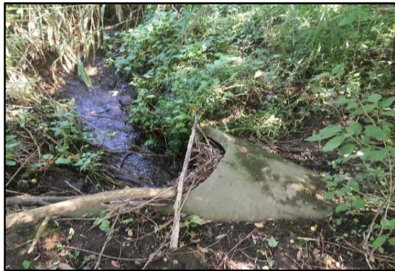
Basin outlet on south side
