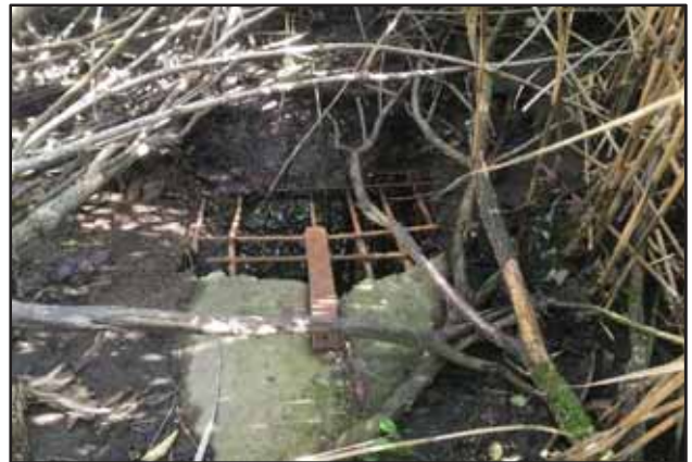
Outlet of storm sewer downstream of basin
