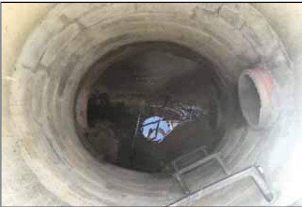
Manhole upstream of detention basin
