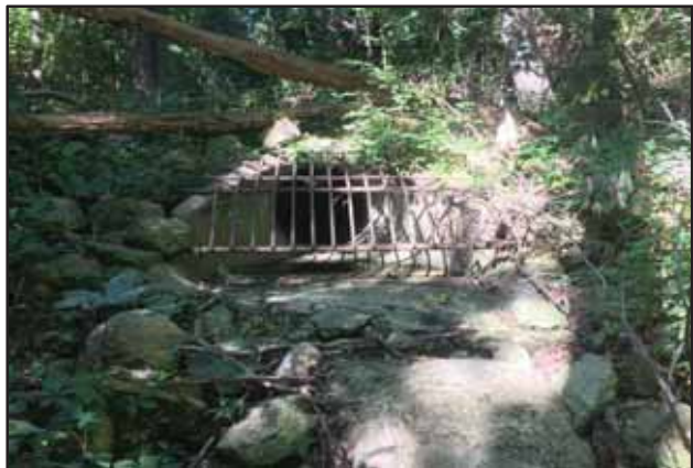
Downstream end of enclosed ditch/sewer
