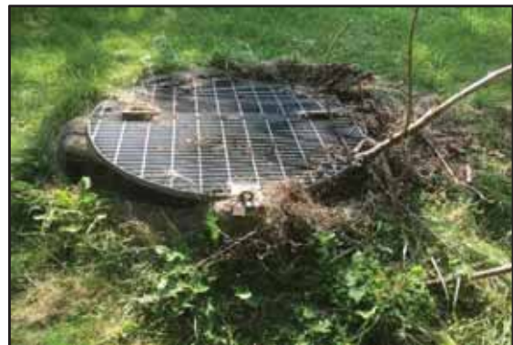
Basin Overflow Structure on south side
