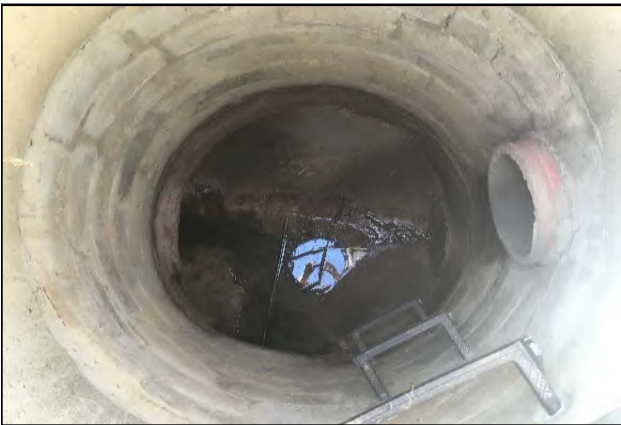
Manhole upstream of detention basin
