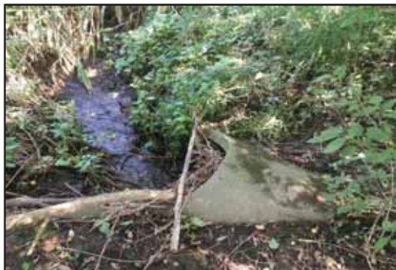
Basin outlet on south side
