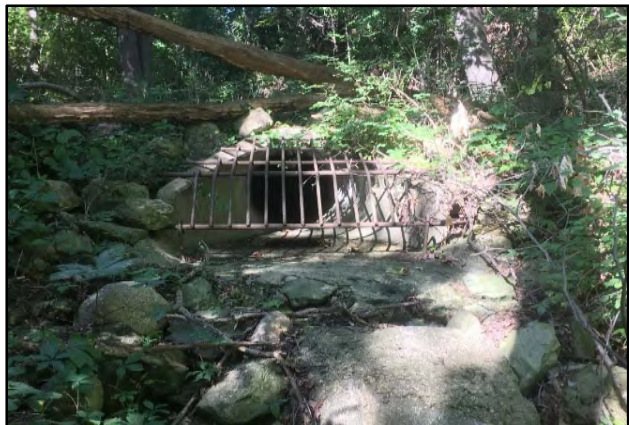
Downstream end of enclosed ditch/ sewer
