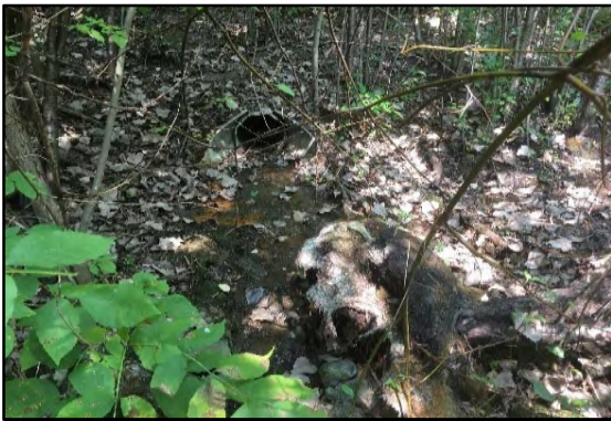
Basin inlet on North side
