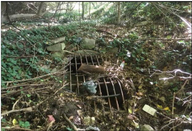
Upstream end of enclosed ditch/ sewer
