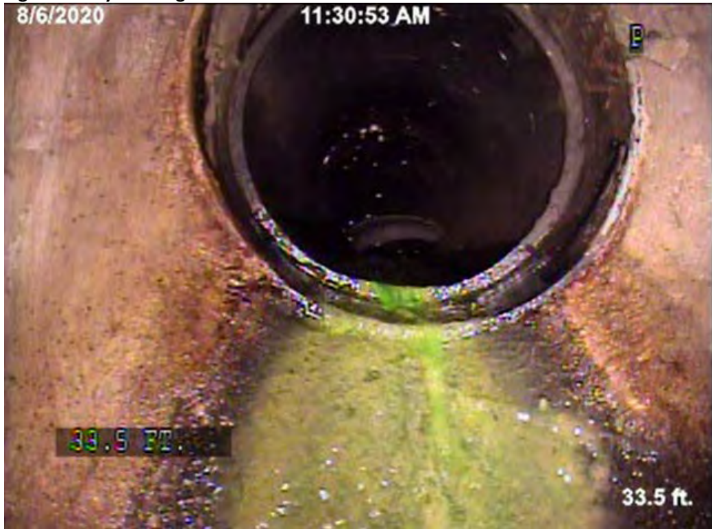
Figure 3C: Dye testing results from basement bathroom
