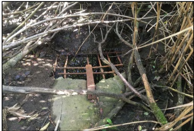
Outlet of storm sewer downstream of basin
