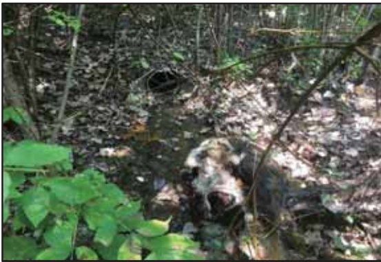
Basin inlet on North side
