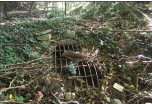
Upstream end of enclosed ditch/sewer
